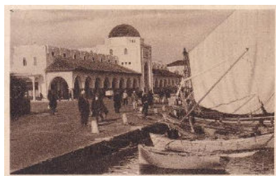
PPC The facade of the market
